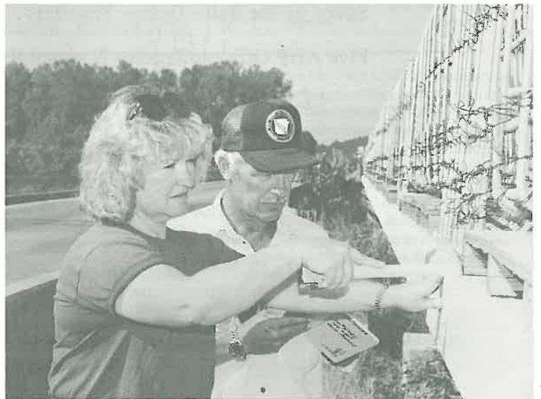
Patti Clowers , Construction Aide III, and Gary Roberts , Senior Inspector for the Texarkana Resident Engineer's Office in District 3, inspect contractor's work on the Highway 41 bridge crossing the Red River south of Foreman.
