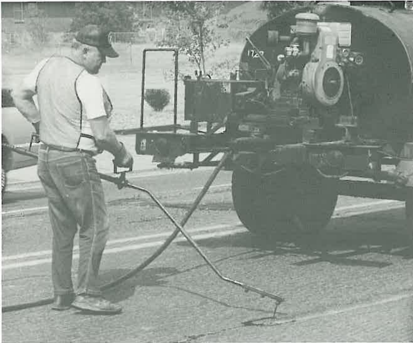
Tom Reed , Motor Patrol Operator/Finish for the District 4 Sebastian II maintenance crew, hand sprays tack prior to a patching operation in preparation for an overlay on Highway 71B in Fort Smith.
